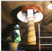
Stonbury were recently commissioned to carry out refurbishment works to the gas zone of a Digester. The inspection to the soffit, revealed that the existing coating had failed and that the exposed concrete had suffered from attack by the Hydrogen Sulphide gases.
