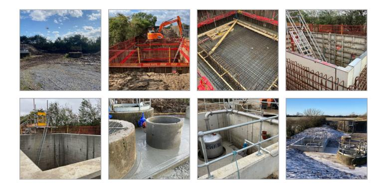
Stonbury constructed a newly built reinforced concrete storm tank and overflow discharge chamber within a Sewage Treatment facility.
