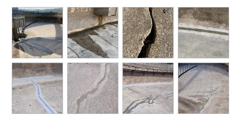
Stonbury was enlisted to complete emergency repairs to a storm tank floor after leakage was discovered through several areas in the floor.
