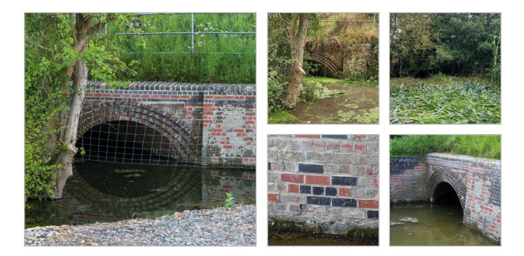
Stonbury was awarded a scheme to carry out brickwork repairs to a 50-metre-long Victorian-built flood alleviation culvert after the railway company completed a structural report and found issues with the brickwork.
